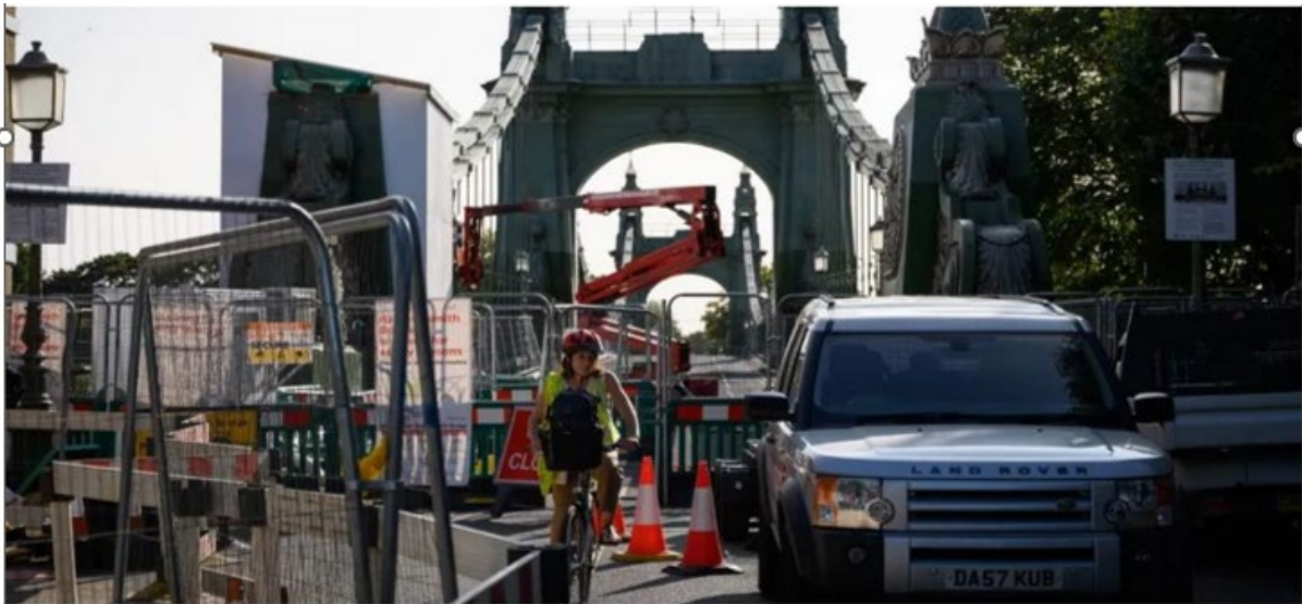
Figure 1: Hammersmith Bridge under repair since 2019
